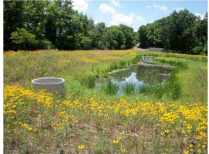
captured stormwater is slowly released to Arcadia Creek over a 48-hour period following each rainfall event. Some fraction of stormwater is also infiltrated to groundwater. Construction for the Lot 23 Stormwater Treatment System began in late July 2009 and was completed in early October 2009.
