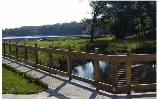
Subsequent performance monitoring by K&A in 2007, revealed 81% removal of TP and 81% removal of TSS loads that would otherwise discharge into Woods Lake. Overall, the system's treatment efficiency for phosphorus is above what was originally designed.
